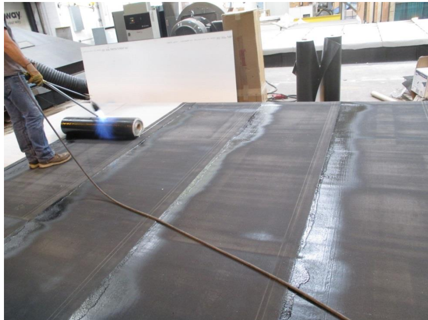
Photo No. 2 Torching the Base Sheet
