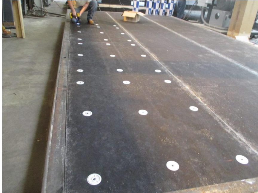
Photo No. 1 IKO Protectoboard over the Wood Sheathing
