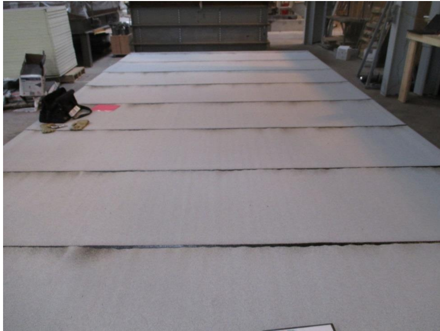
Photo No. 3 Finished Cap Sheet
