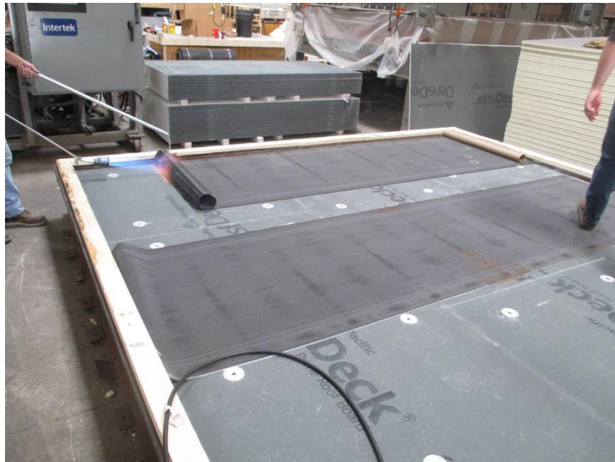
Photo No. 2 Vapor Barrier
