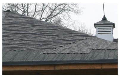
Conventional organic felts can absorb moisture, causing severe buckling and wrinkling—and a terrible-looking roof
