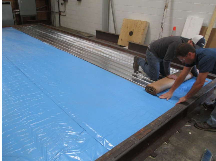
Photo No. 3 Vapor Shield
