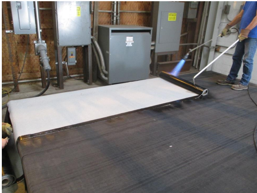
Photo No. 6 Self-Adhered Base Sheet and Torched Cap Sheet
