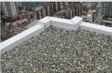
Protected / Ballasted Roofs
