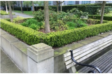
Waterproofing Systems & Planters
