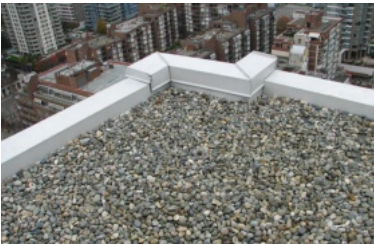
Protected / Ballasted Roofs
