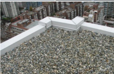
Protected / Ballasted Roofs
