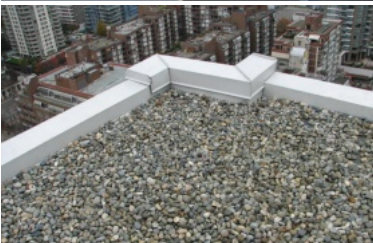
Protected / Ballasted Roofs
