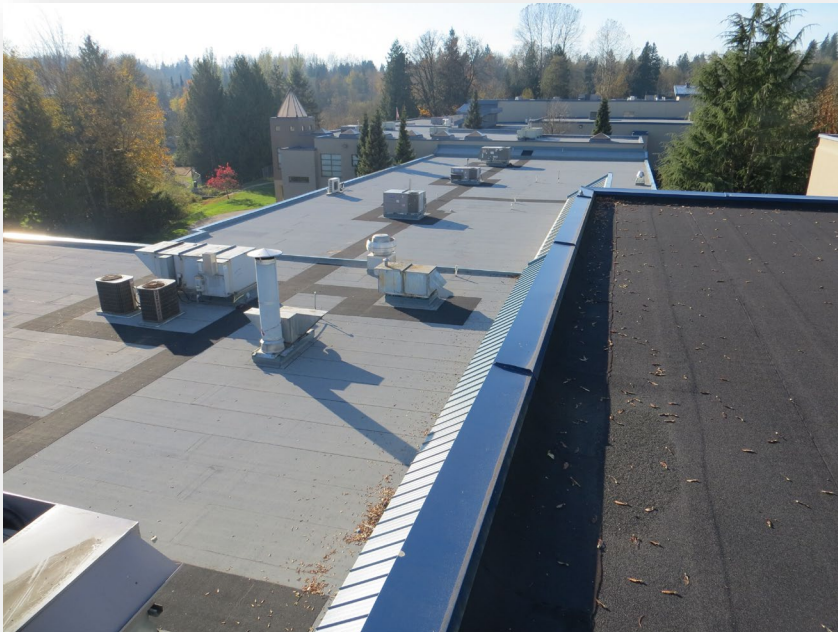
Membrane roof (SBS-modified bitumen)
