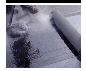
When used with a cap sheet, IKO **PrevENt MP-HD-Cap** Fully Adhered Cap Sheet satisfies the requirements of CGSB-37.56-M, as well as ASTM D6162 for Type I, Grade G materials. It also qualifies for a Class A rating in accordance with CAN/ULC S107M and UL790 test protocols.
